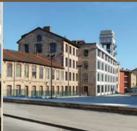
3. "Lanificio Conte" Wool Mill and Conte Square
