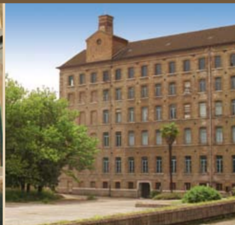
4. "Fabbrica Alta" Factory
